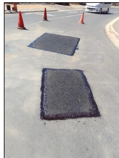
FIGURE 50: POTHOLE PATCHING
